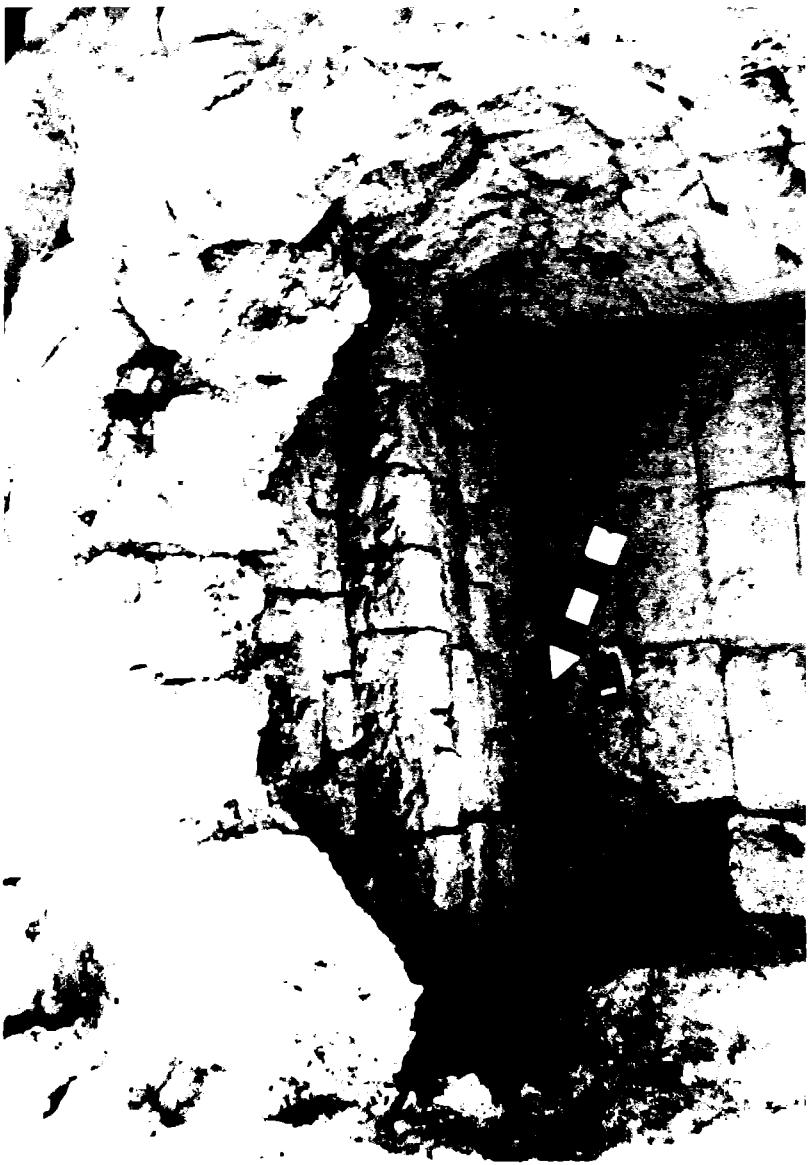
16. Clay brick construction—Assyrian type, 7th cent. B.C.E., Tel-Jemme. Israel Exploration Society.
